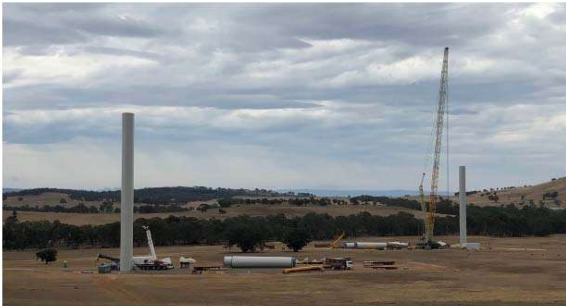
Figure 2 – Pre-Installation at BU01 & BU01 in Collector Group 1
