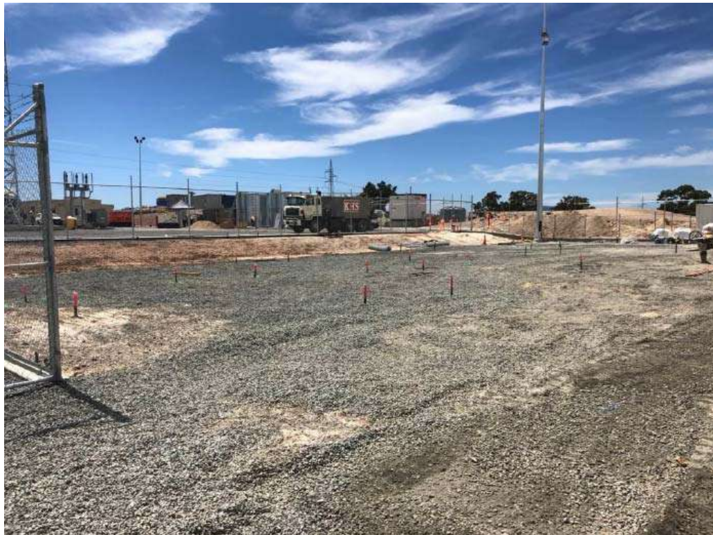
Figure 5 – BESS Bench Preparation
