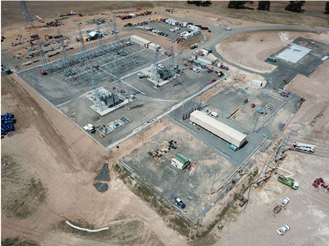
Figure 3 – Terminal and Substation Progress
