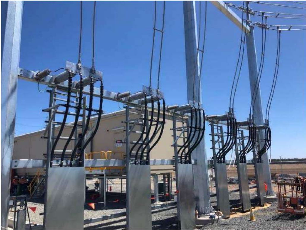
Figure 4 – Overhead Gantry and Droppers Progress
