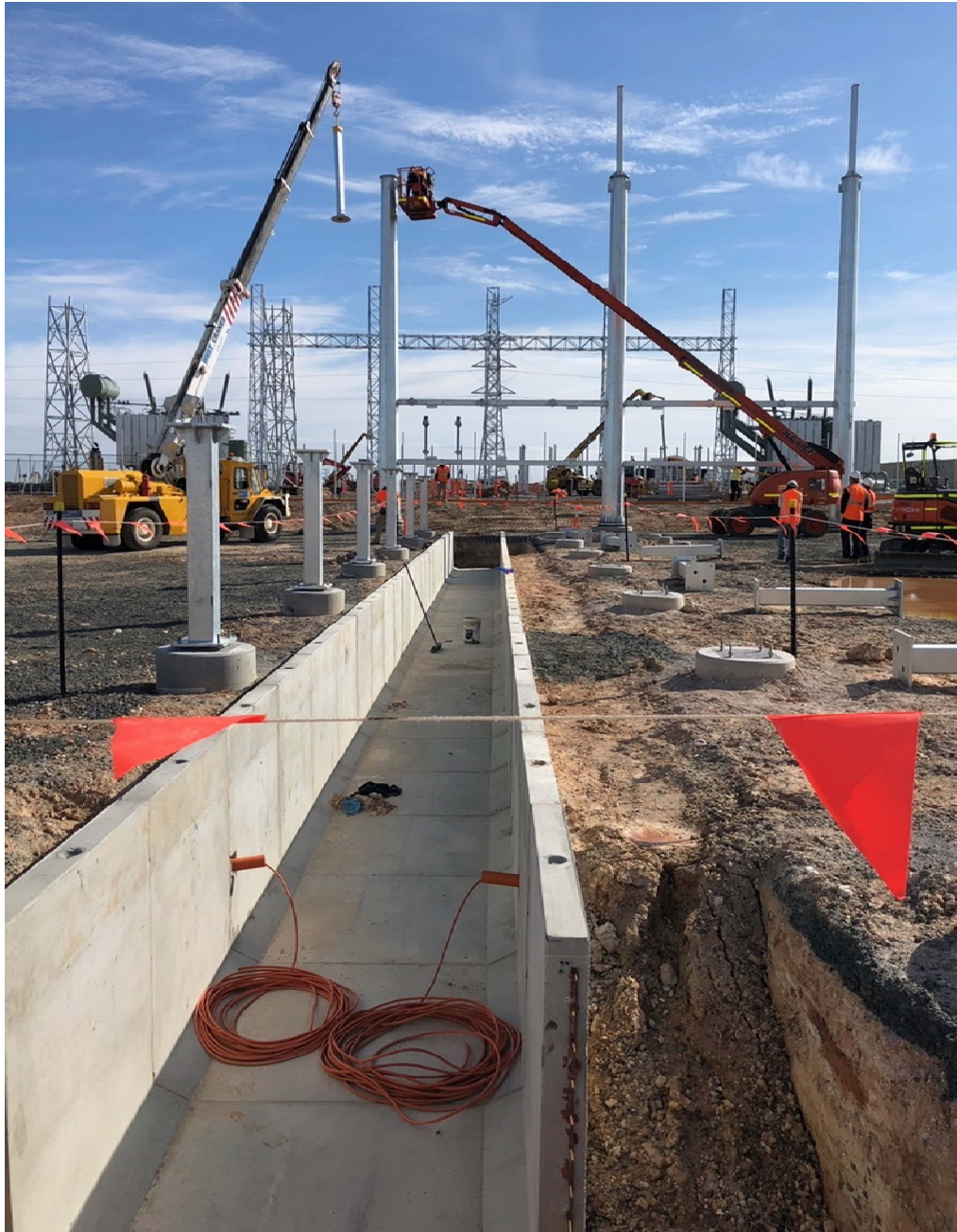
Figure 3- Switch room Culvert & Foundation Works and Gantry Installation at background
