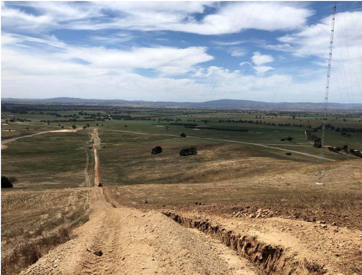
Figure 5 – U/G Cable Trenching Work for POLE 53 Up to BU23
