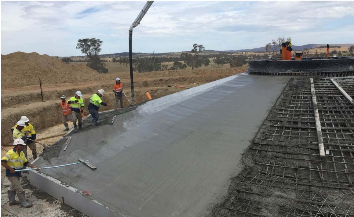
Figure 4- Main Concrete Pour at BU59
